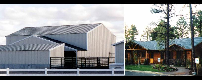
The Perma-Clad® panel system can be used for both roof and wall applications. Perma-Clad® is great for residential, light commercial, agricultural and storage buildings and also for canopies. The Perma-Clad® panel must be installed over a solid, waterproofed deck when used as a roof panel.
