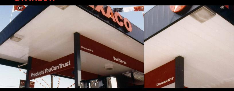
QwikLok<sup> $\mathbb{M}$ </sup> is ideal for underhung applications. No more fighting with trying to install two panels at one time. Unlike conventional roofing cover, QwikLok<sup> $\mathbb{M}$ </sup> can be assembled from the underside of the structure one panel at a time, producing a flush appearance with no exposed fasteners.
