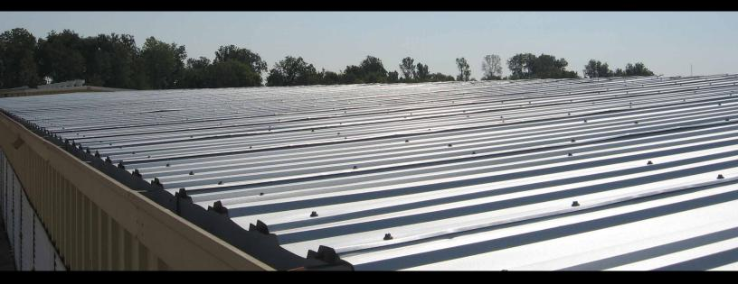
The Retro-R® Panel is an excellent choice for retrofit construction, and can be applied directly over an existing PBR or R panel to give your building a new look and longer life. This exposed-fastened system has a membrane on the back side to prevent rust from the old roof and from transferring to the Retro-R® panel.
