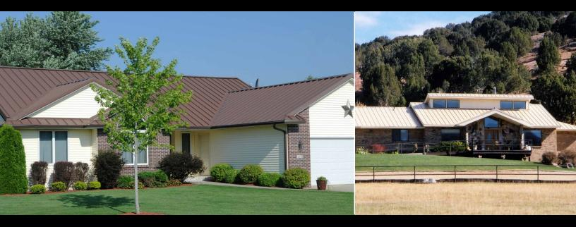
The Slimline® roof panel system offers a sleek contemporary profile ideal for residential and light commercial applications. This system offers a concealed fastener attachment. Slimline® panels must be specified as striated or striated with minor ribs. Slimline® cannot be endlapped.
